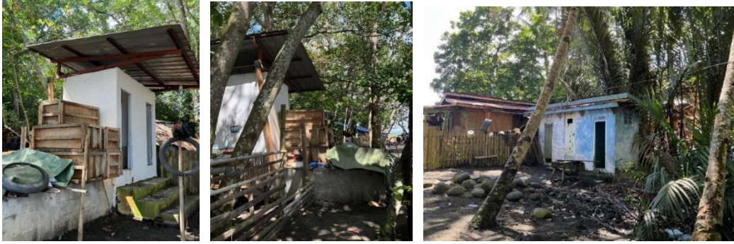
Figure 8. Anthropogenic Infrastructure: Documentation of residential septic tanks and comfort rooms adjacent to the high-tide mark, indicating risks of fecal leaching.
